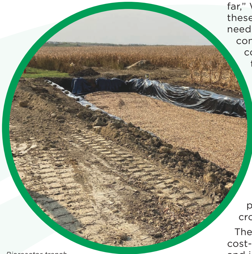
Bioreactor trench with wood chips for Farm to River project.
